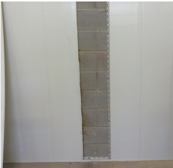
Figure 6 Remove damaged panel
