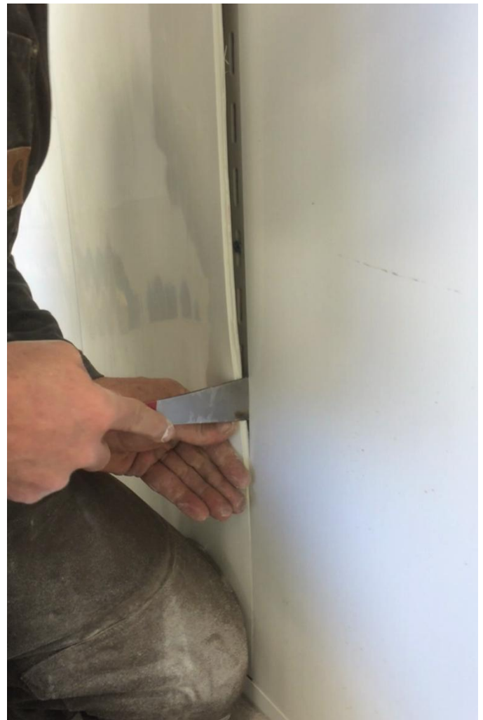
Figure 13 Pry the interlocking edge into adjacent panel
