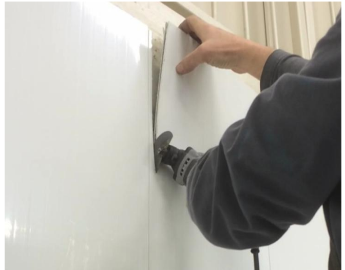
Figure 3 Begin cutting the panel
