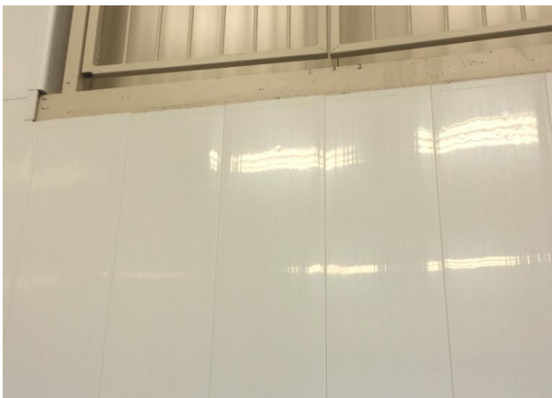
Figure 2 J-Trim removed from top of panels
