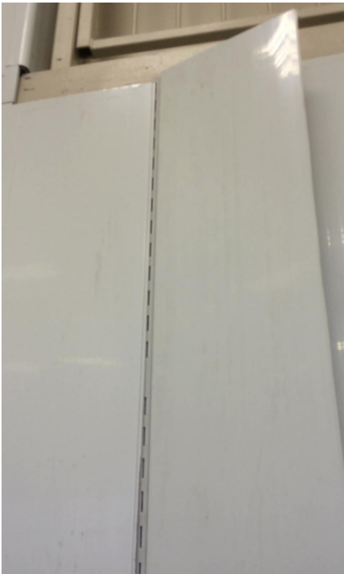
Figure 12 Insert nailing strip into adjacent panel
