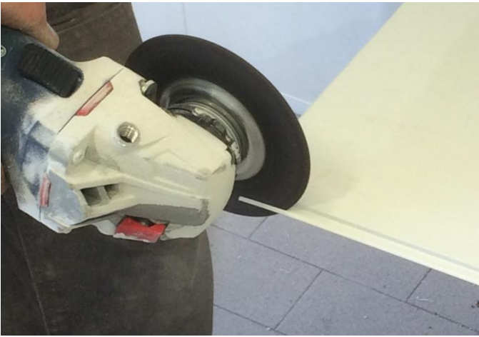
Figure 9 Trim lip of interlocking edge
