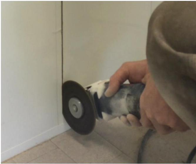
Figure 5 Stop cutting just above trim to avoid damage
