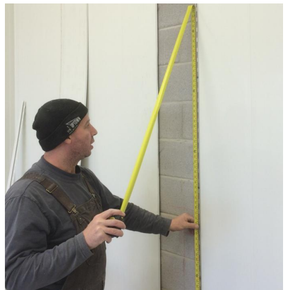
Figure 8 Measure required length of new panel
