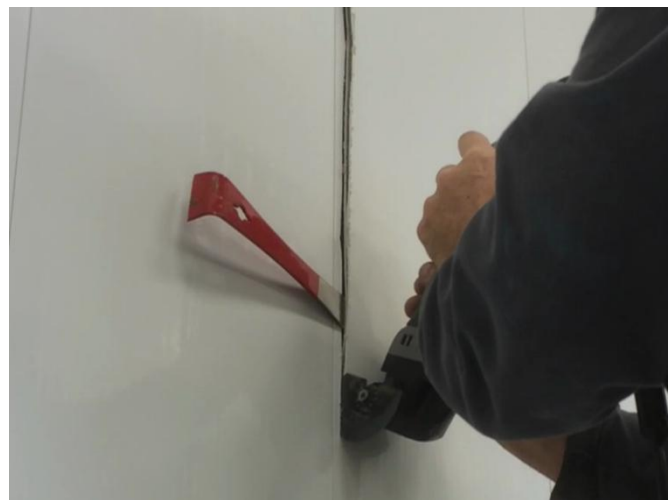
Figure 4 Use scraper bar to pry panel away from wall
