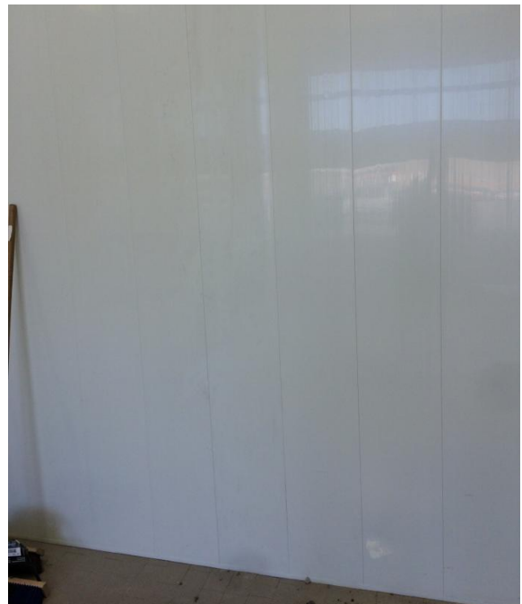
Figure 15 Completed panel replacement
