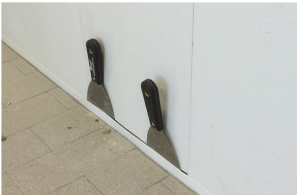
Figure 14 Scrapers help guide the panel into the trim
