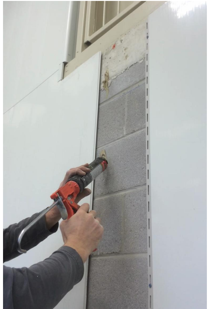
Figure 11 Apply adhesive
