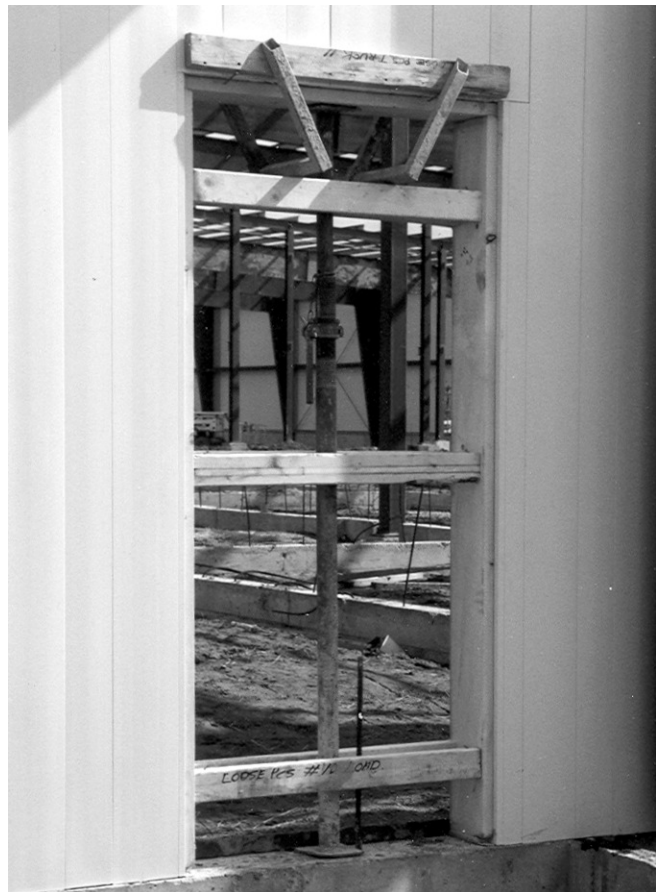
11.6c Bracing at Door Opening
