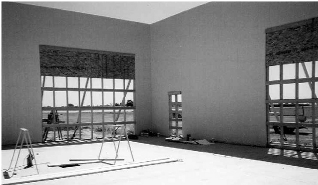
7.6c Bracing of Openings
