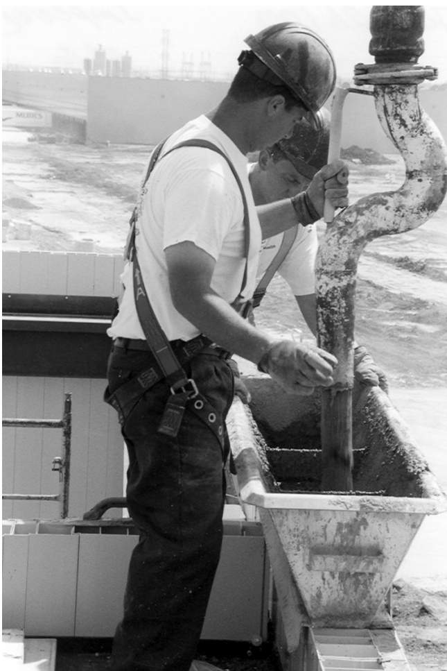
12.1b Concrete Funnel, Reducer and S-Bend
