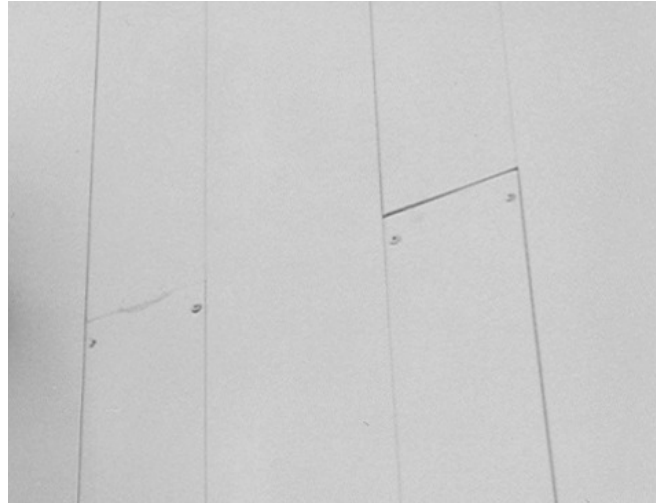
9.1b Screws at Staggered Joint
