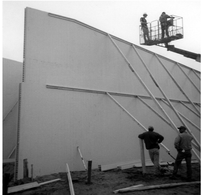
11.3a Mid Height Bracing at One Side
