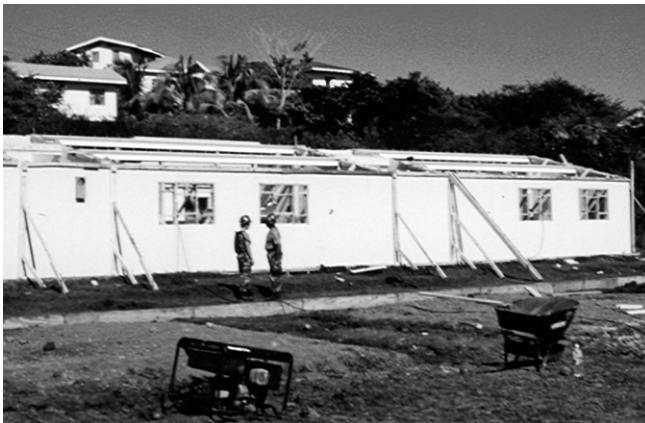
11.5c Bracing at Wall Intersection
