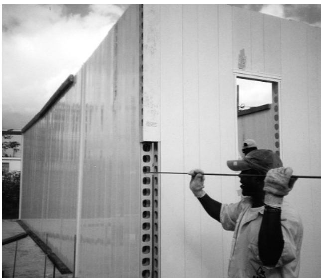
10.1b Horizontal Reinforcing Bars
