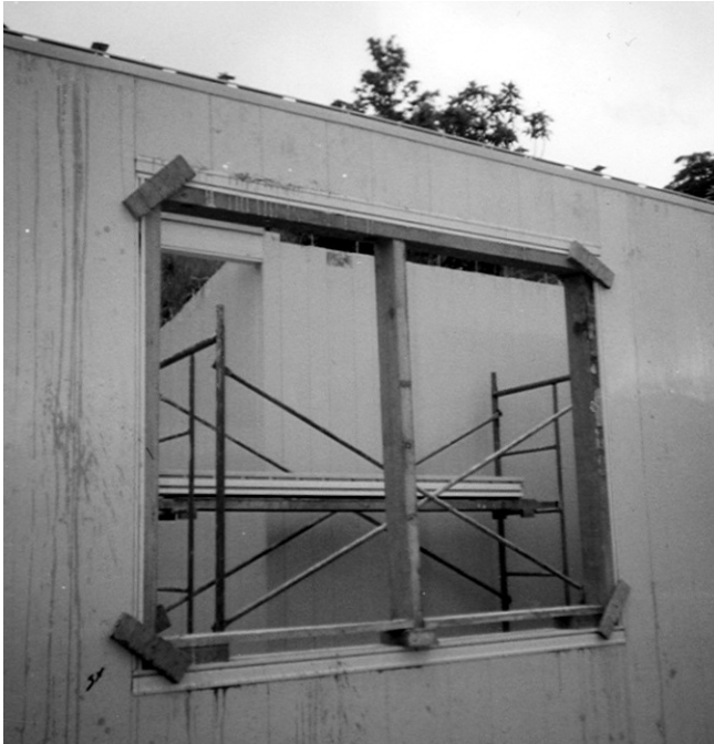
11.6a Bracing at Opening
