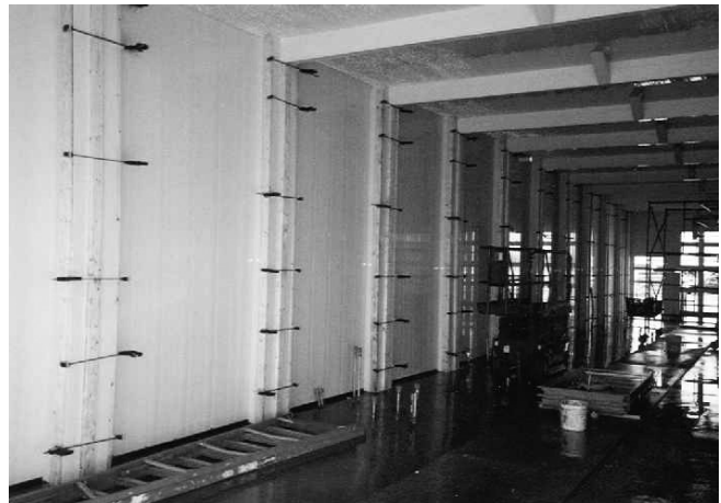
11.5d Bracing at CONFORM Pier
