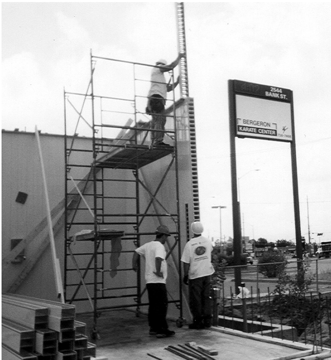
8.2b Erection of CONFORM
