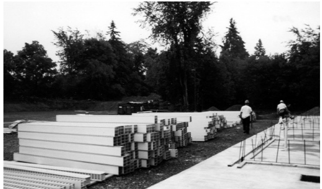
6.2a Storage of Individual Components
