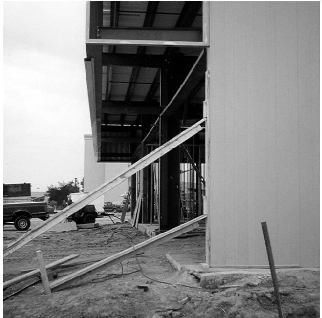
11.5a Bracing at End of Wall
