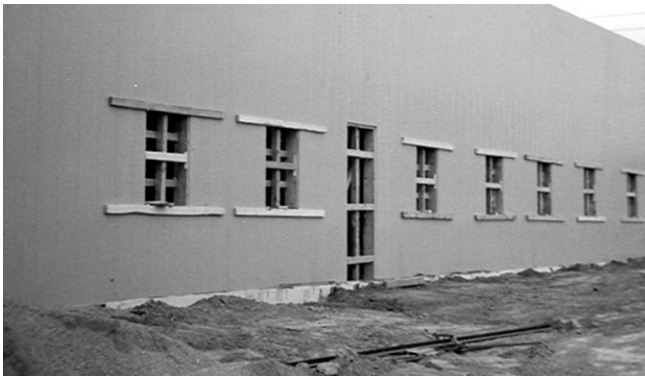
11.6b Bracing at Window Opening
