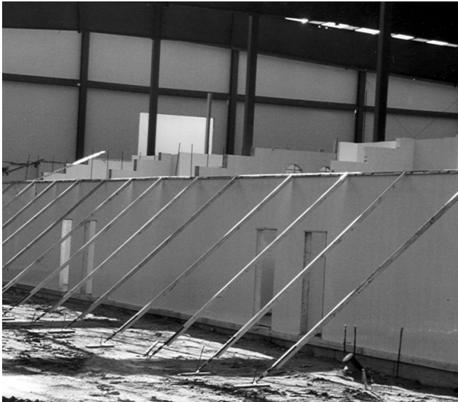
11.4a Top Bracing at One Side
