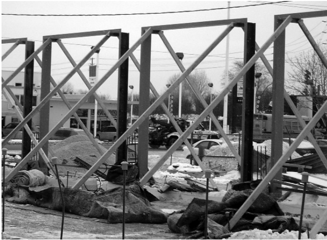
7.6a Overhead Door Frame Installation
