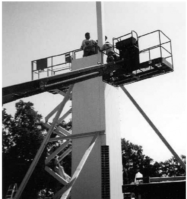
8.2a Erection of CONFORM Corner
