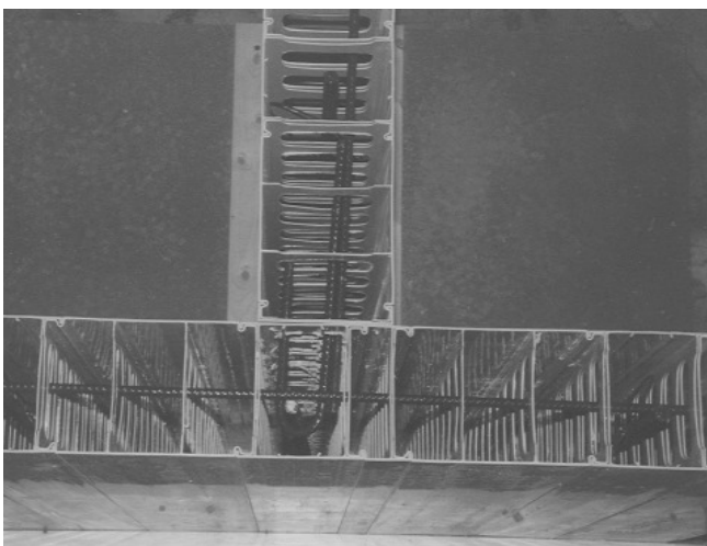
10.2b Intersection Hooked Horizontal Bar
