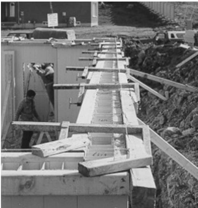
11.4b Top Bracing at Both Sides
