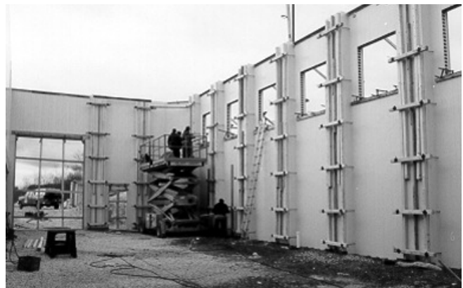
11.5e Bracing at High Pier
