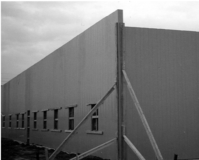
11.5b Bracing at Corner
