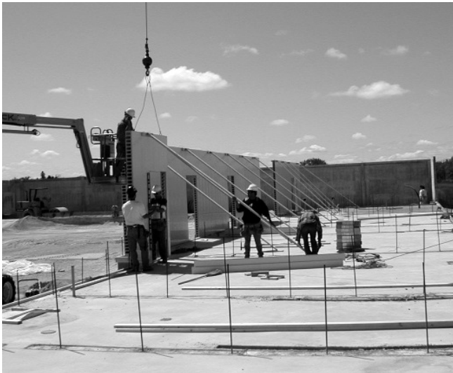
9.1c Pre-assembled Wall Section Lowered over Dowels
