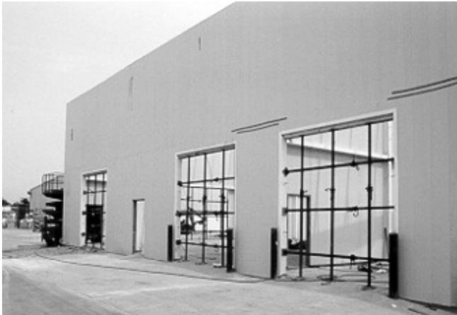
11.6d Bracing at Overhead Door
