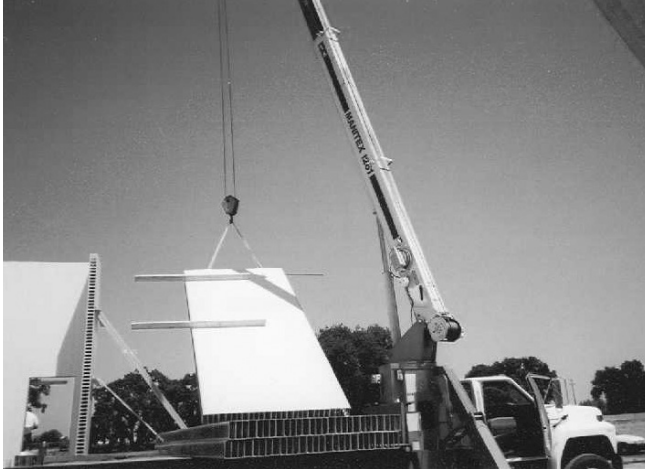
6.2b Storage of Pre-assembled Wall Sections
