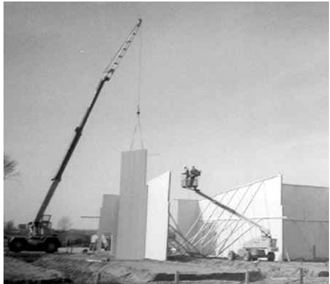
2.4b Erection of Pre-assembled Wall Section
