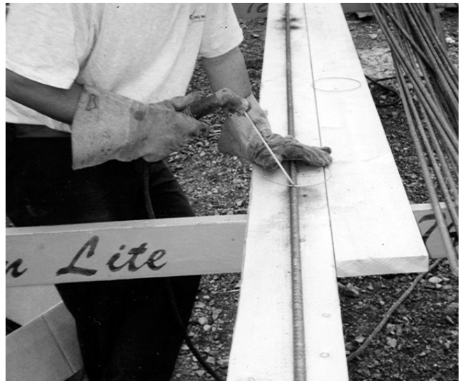
3.3 Vertical Rebar with Hoop
