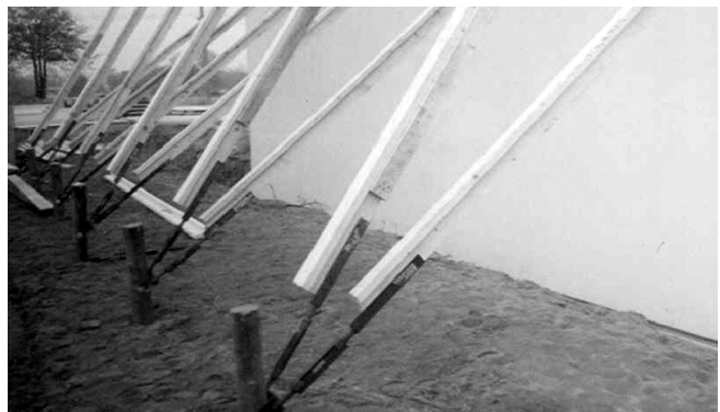
7.3 Wall Bracing and Form Aligners
