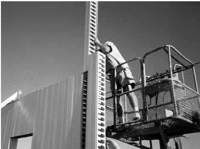
8.1 Erection of CONFORM® Box and Panel
