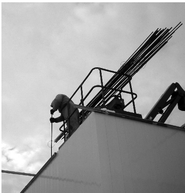
10.1a Vertical Reinforcing Bars
