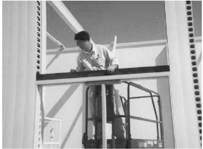
7.6b Steel lintel Installation
