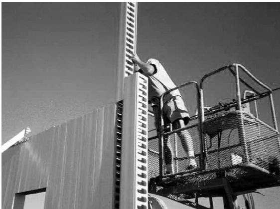
8.1 Erection of CONFORM® Components
