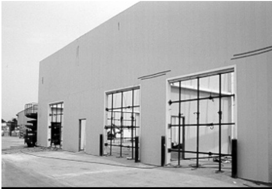
11.6d Bracing at Overhead Door
