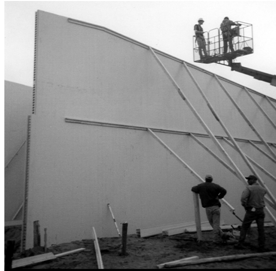
11.3a Mid Height Bracing at One Side
