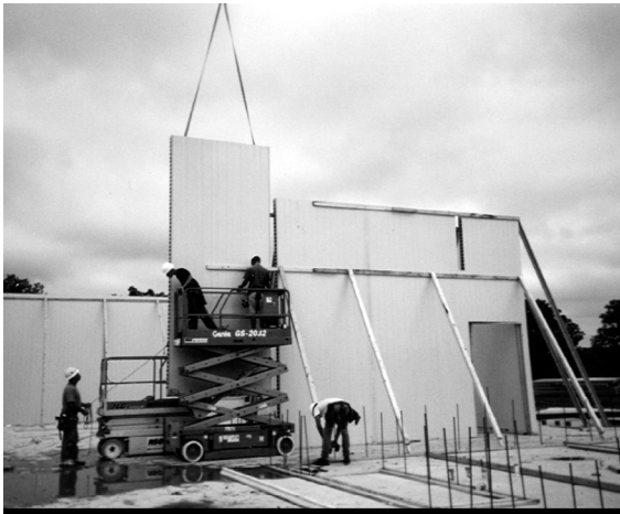
9.1a Erection of Pre-assembled Wall Section
