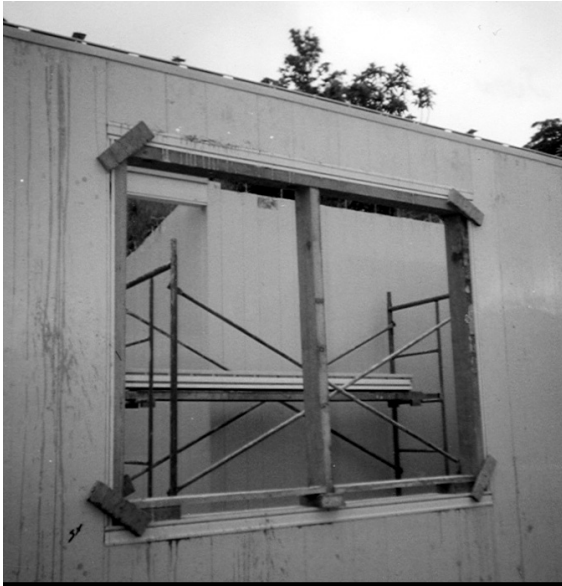
11.6a Bracing at Opening
