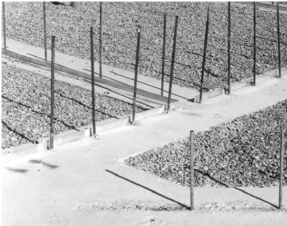
7.2 Metal Strapping and Dowels
