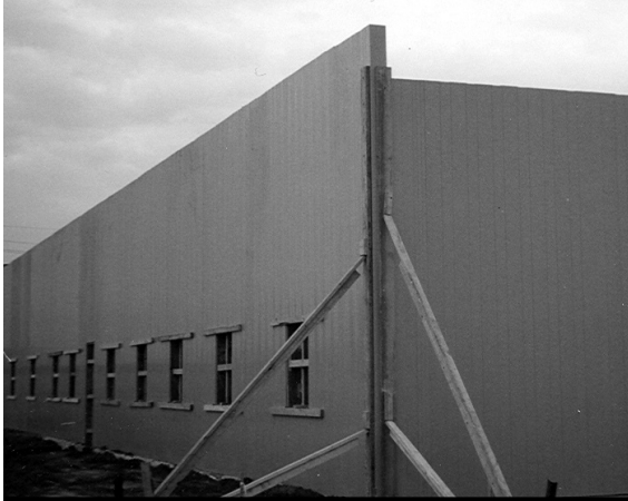
11.5b Bracing at Corner
