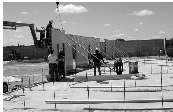
9.1f Pre-assembled Wall Section Lowered over Dowels
