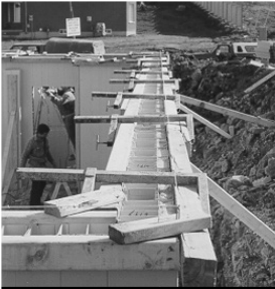
11.4b Top Bracing at Both Sides
