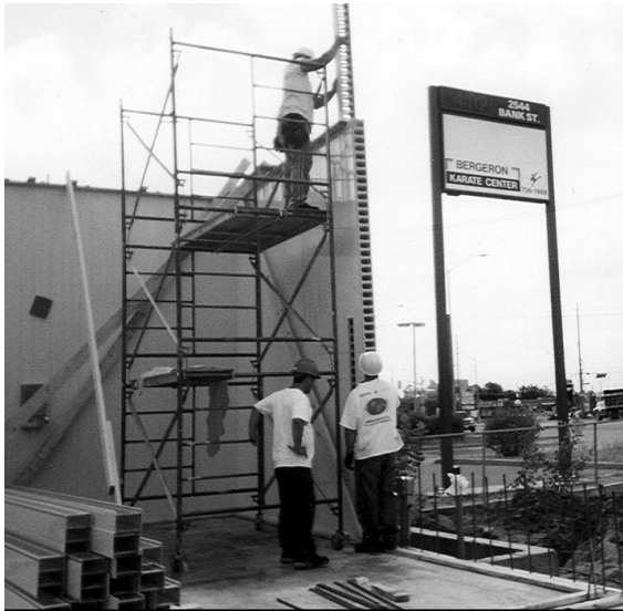
8.2d Erection of CONFORM® Components
