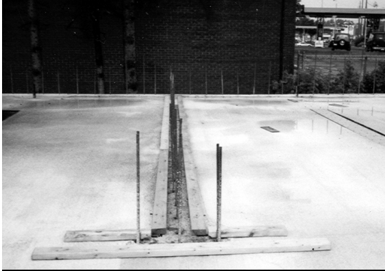
11.2b Bottom Bracing at Both Sides
