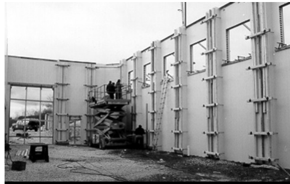
11.5e Bracing at High Pier
