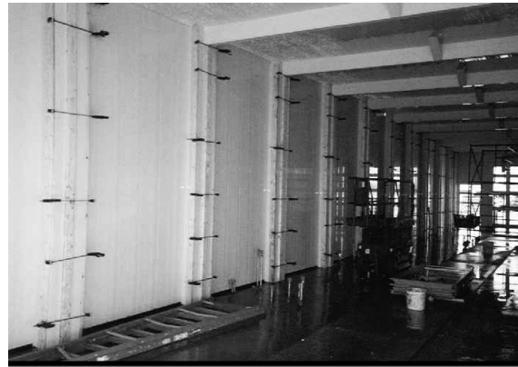
11.5d Bracing at CONFORM Pier
