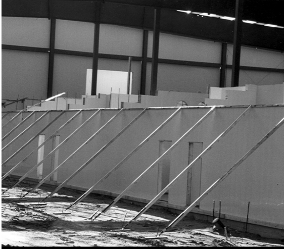
11.4a Top Bracing at One Side
