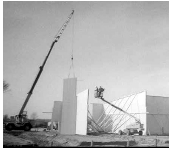
2.4b Erection of Pre-assembled Wall Section
