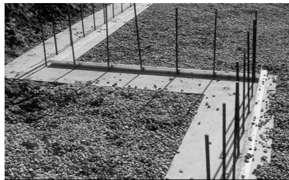
11.2a Bottom Bracing at One Side
