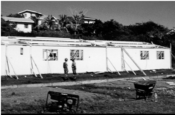
11.5c Bracing at Wall Intersection
