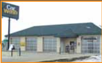
Self-Serve & Automatic Building
