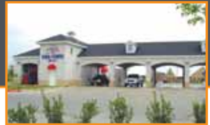
Self-Serve & Automatic Building
