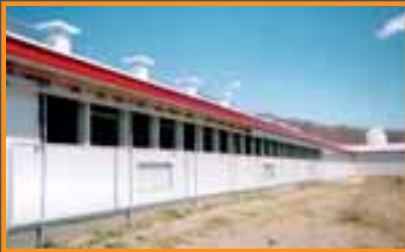
Natural Ventilation Barn
