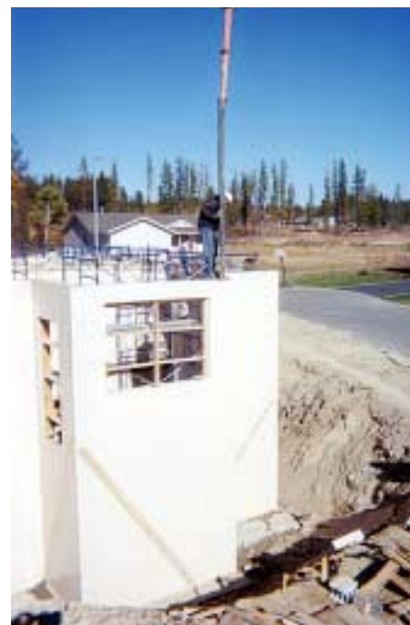
Vancouver home builder Dan Webster completes walls with concrete-filled polymer components
