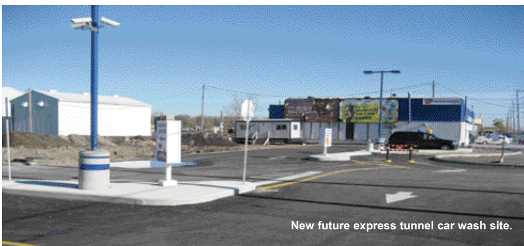
Eight-bay self-serve car wash structure.
