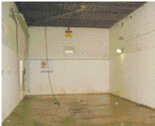
Seven-bay self serve before retrofit.
