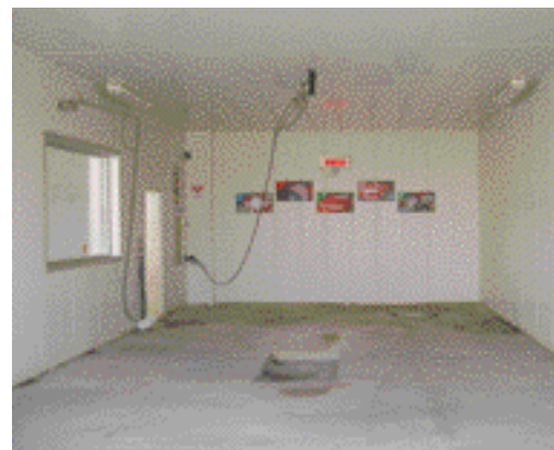
Seven-bay self serve after retrofit.
