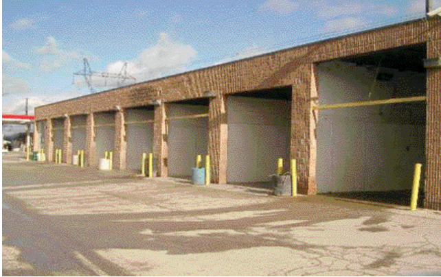
Seven-bay self serve before retrofit.
