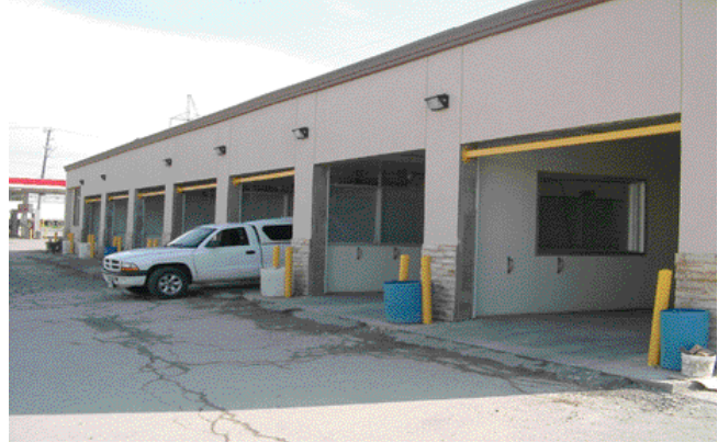
Seven-bay self serve after retrofit.
